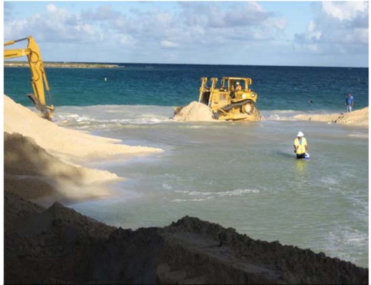
Figure 28 The City uses heavy equipment to open the stream mouth about nine times per year.
