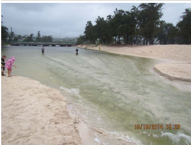
Figure 30. October 2014 the City responded to a high water surface in the pond and an impending rainstorm to conduct an “emergency” opening of the stream mouth. Flow established in a 1-foot deep 15 foot wide channel completed at 16:15 developed into a 30-foot wide 3 foot deep channel in about an hour and fifteen minutes. Within minutes of the last photo the cameraman had to abandon his location as the bank was eroding from beneath his feet.
