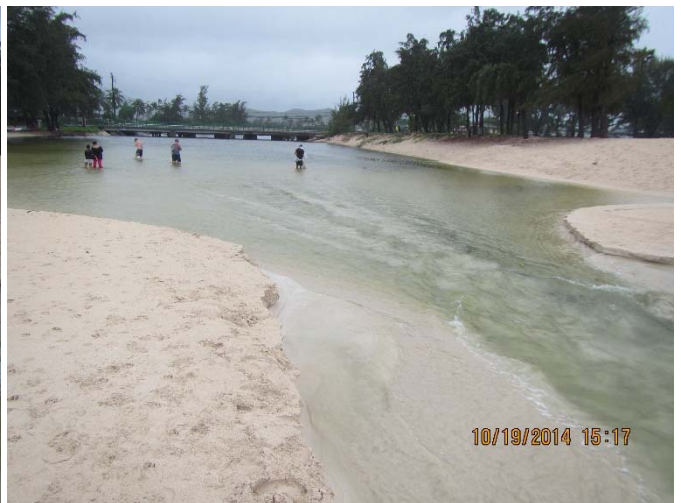
Figure 30. October 2014 the City responded to a high water surface in the pond and an impending rainstorm to conduct an “emergency” opening of the stream mouth. Flow established in a 1-foot deep 15 foot wide channel completed at 16:15 developed into a 30-foot wide 3 foot deep channel in about an hour and fifteen minutes. Within minutes of the last photo the cameraman had to abandon his location as the bank was eroding from beneath his feet.
