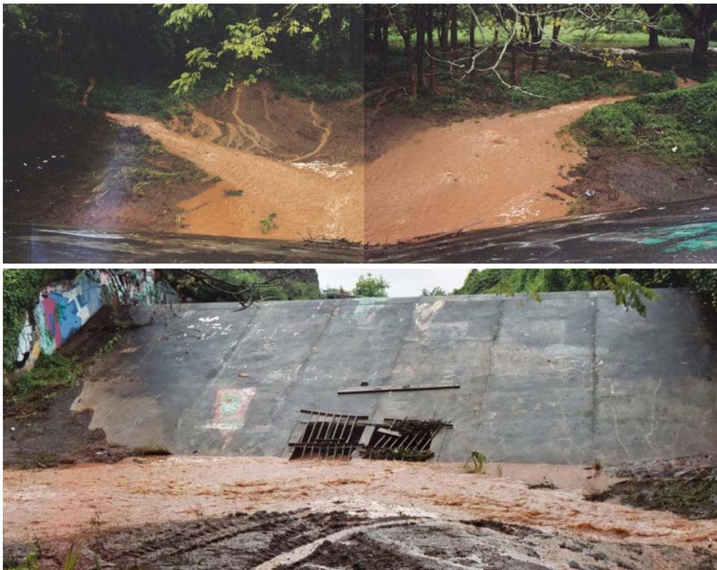
Figure 26. Top: Looking down the inside dam face as muddy water pours through the two erosional channels cut through the internal raised berm. Bottom: Inside the basin looking at the back of the dam face with the muddy water flowing into the two flow control structures beneath the dam.
